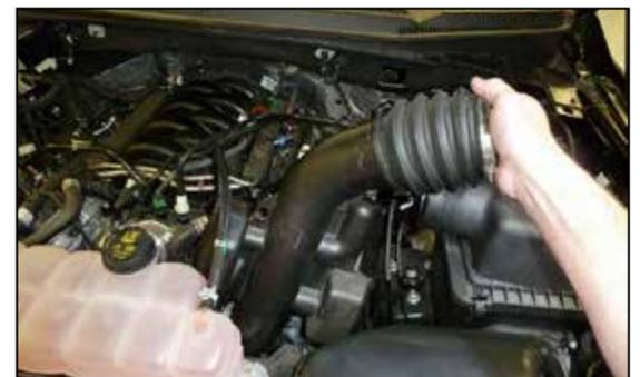
5. Remove the factory intake tube from the vehicle.
