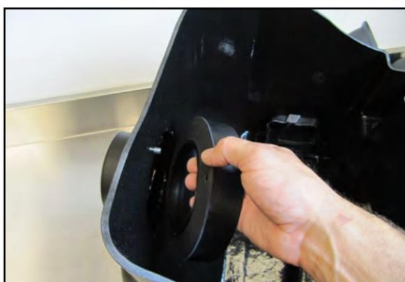
8. Mount the filter adapter and gasket inside the Cool Air Box as shown using the three sets of 1/4-20 button head screws and 1/4" flat washers.
