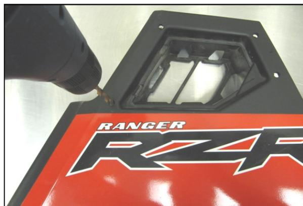
**6.** Using a 9/32" bit, drill out the pilot holes.
