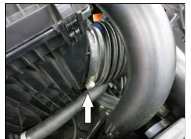
3. Loosen the hose clamp that secures the fresh air duct to the air filter housing.
