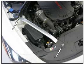
2. Remove the two bolts that secure the passenger side strut tower brace and then remove the brace from the vehicle.
