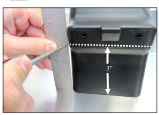
**7.** Set the factory air scoop on a workbench and mark all four corners at the three inch mark using a scratch awl. Using a straight edge and the awl, scribe a line connecting all four corners.
