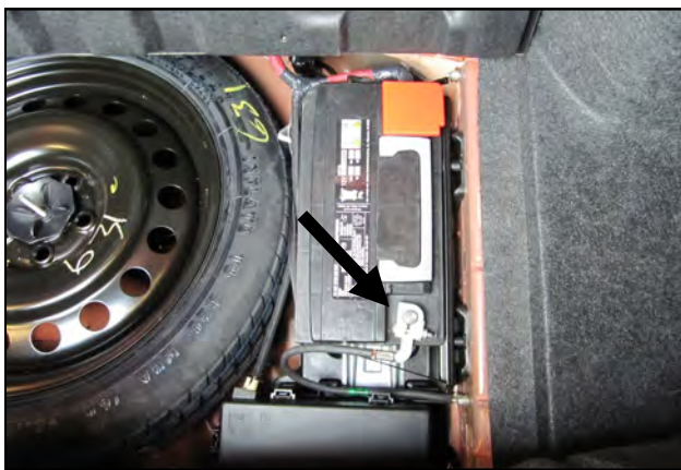
1. Disconnect the negative battery terminal, located in the trunk, by the spare tire.
